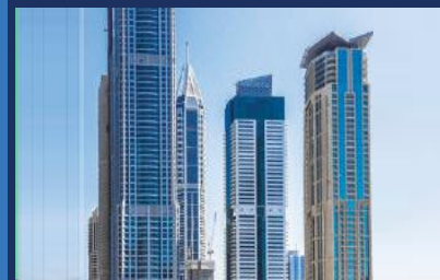
High Rise & Steel Structures
